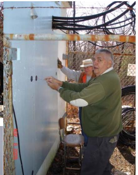
Above: Jim, KC2OGK, fastens insulating panels to the walls of the repeater shack.
